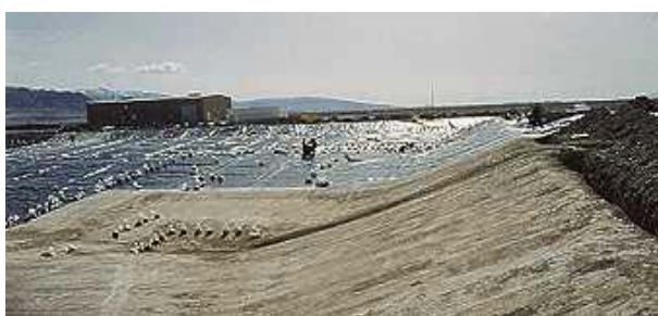
Figure C-5. Clive, UT Mixed Waste Liner Placement
