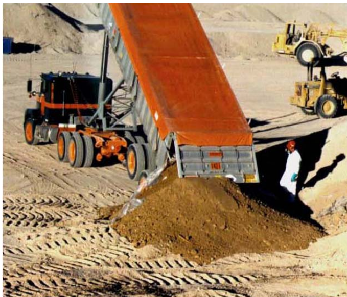
Figure B-12. Disposal in Cell 11, Beatty
