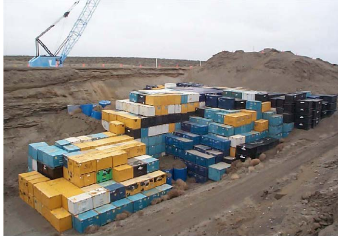
Figure C-9. Hanford, WA Unlined Operating Trench 18
