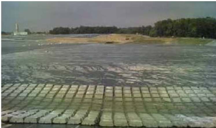
Figure C-29. Maxey Flats, KY Articulated Concrete Block in Drainage
