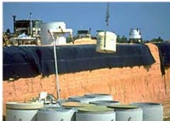
Figure C-14. Barnwell, SC Concrete Vault Placement
