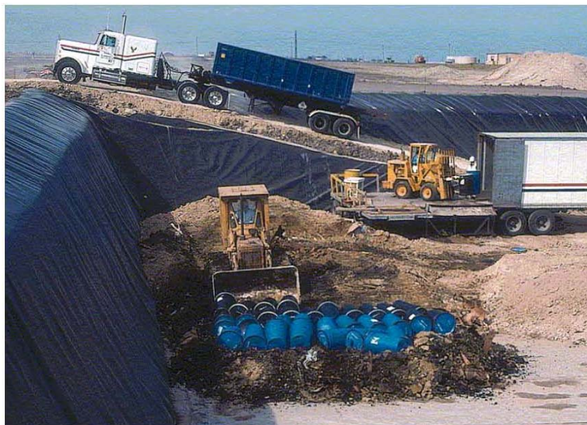
Figure B-16. Disposal at Robstown
